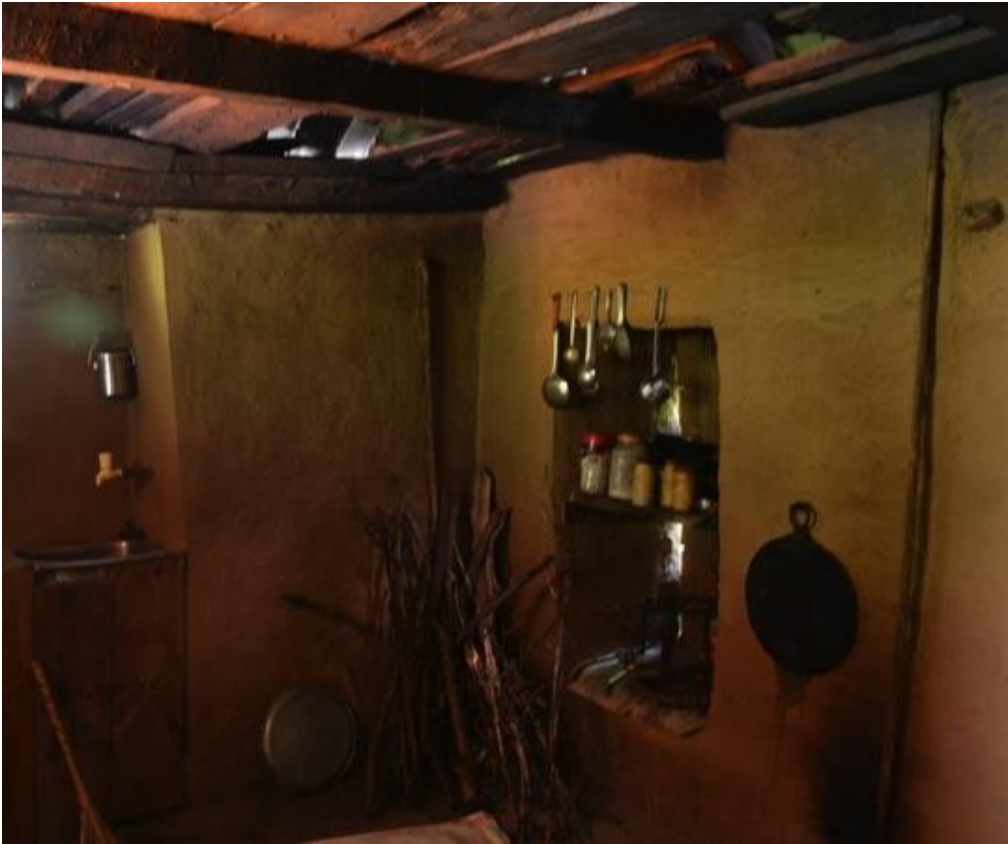
Ceiling opening for House #2 – Roprigad Village:
