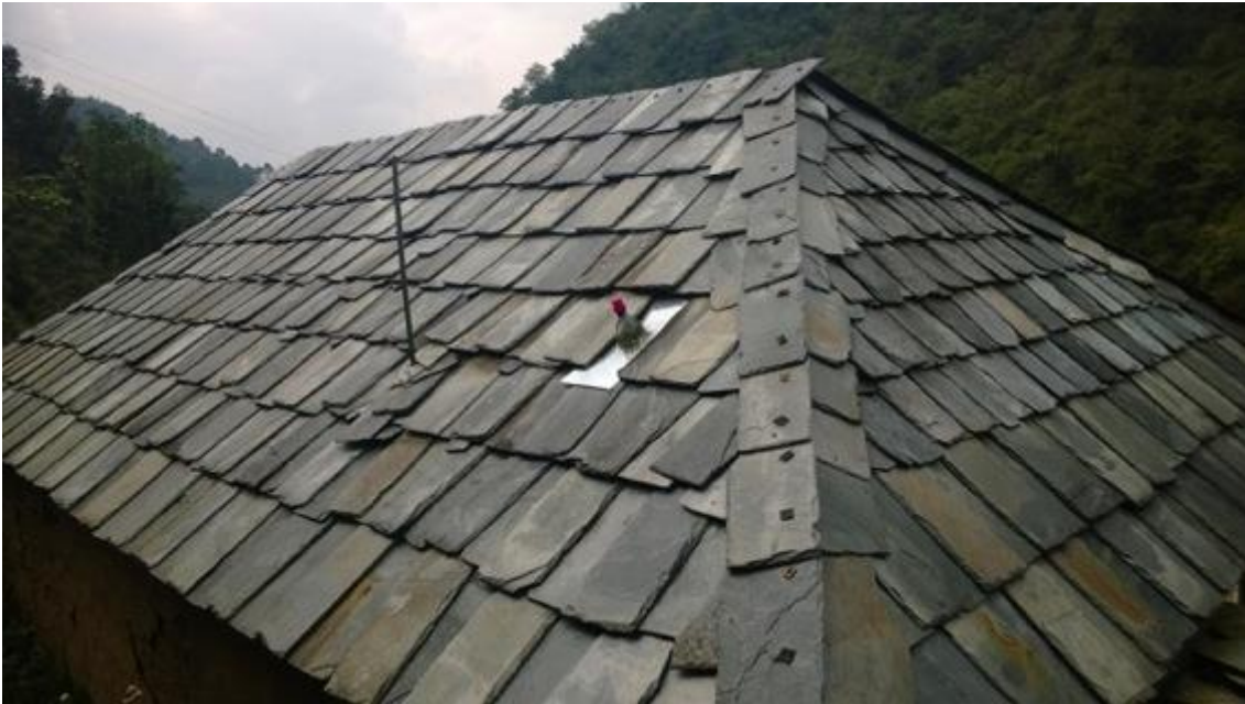
(Outside view of the implemented solar bottle cone prototype)
