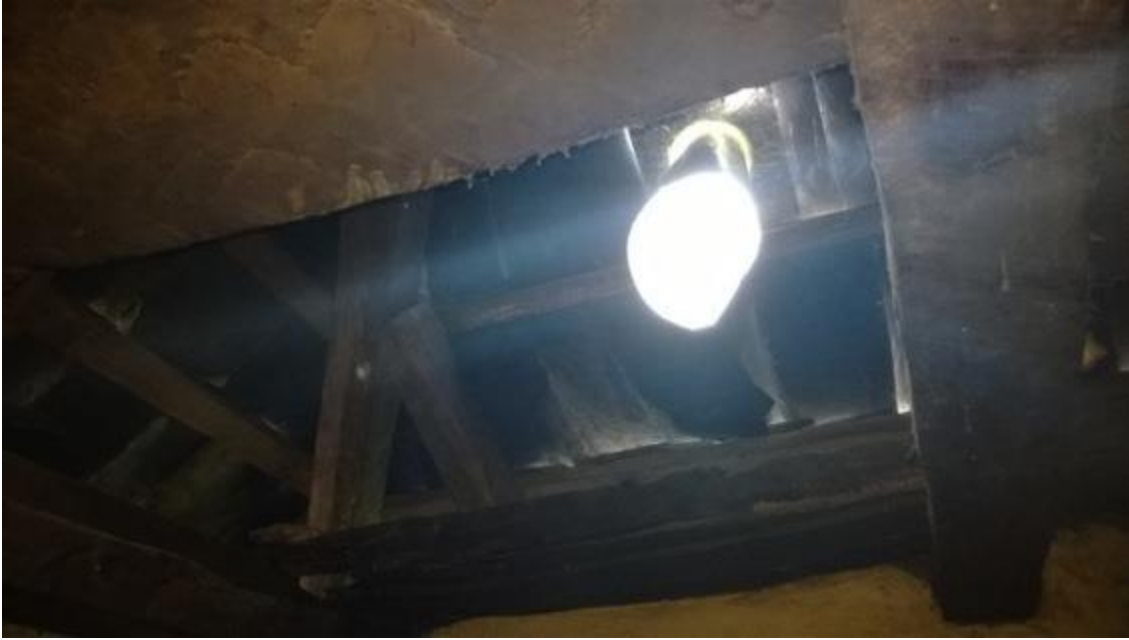
(Photo of the implemented solar bottle cone from the inside of the kitchen)
