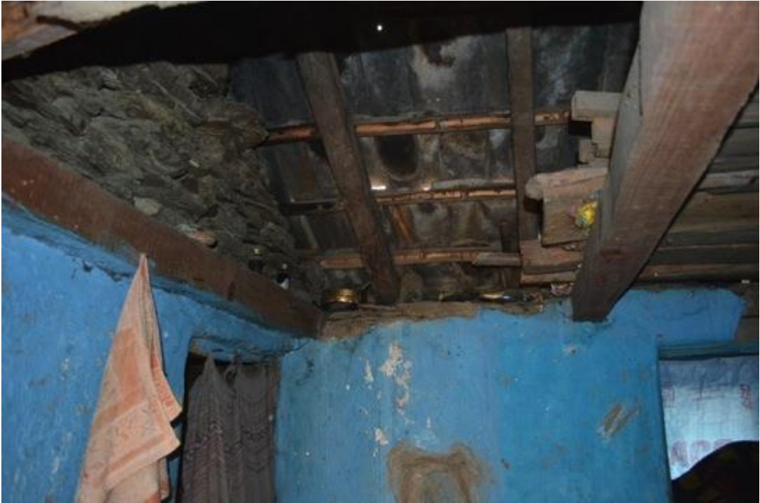
Ceiling opening for House #3 – Fadle Village:
