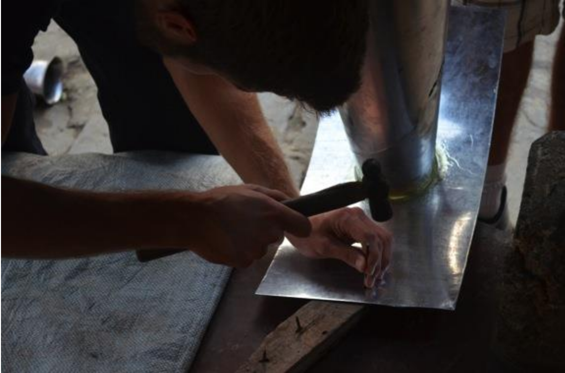
(Photo of team member Mert Can Erad hammering the nail hole)
