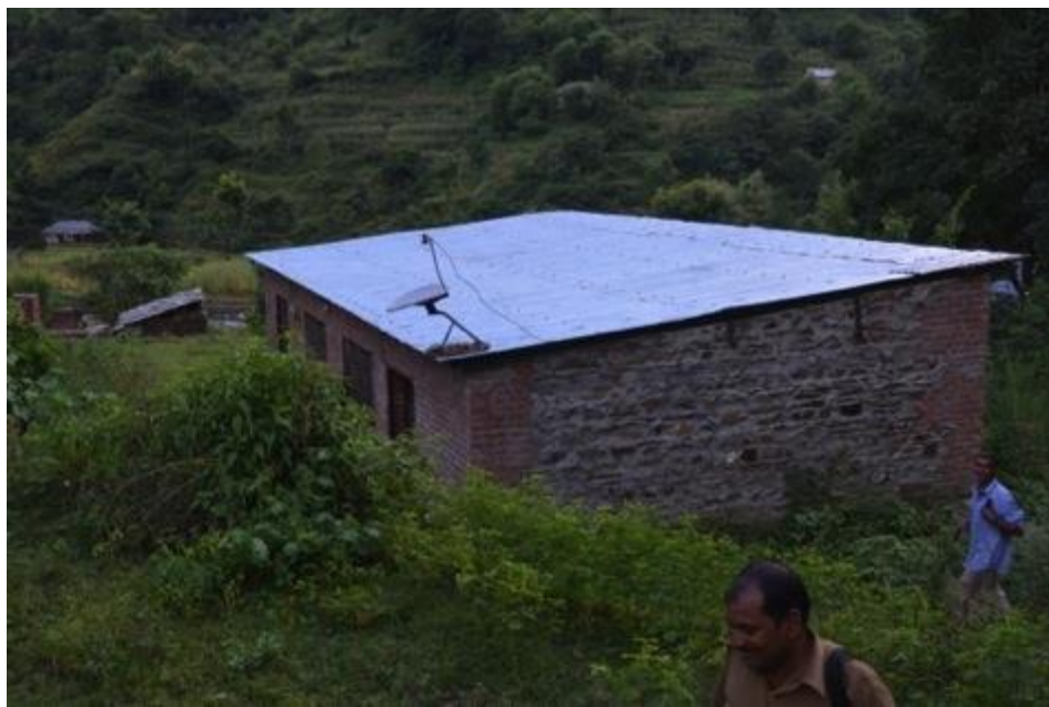
Figure 25: Tin roofed house in Nehri Village (Photo credit: Nehir Keskin, 2013)
