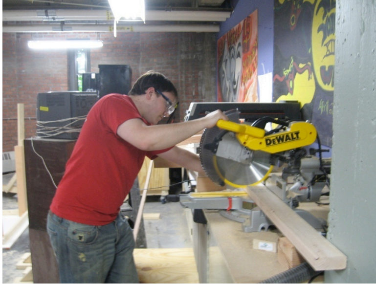
Paul cuts wood with the new chopsaw.
