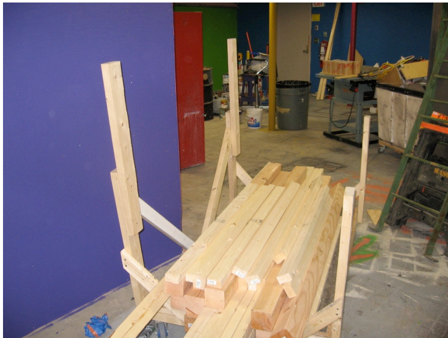
Me used a makeshift cart for moving platforms and lumber.
