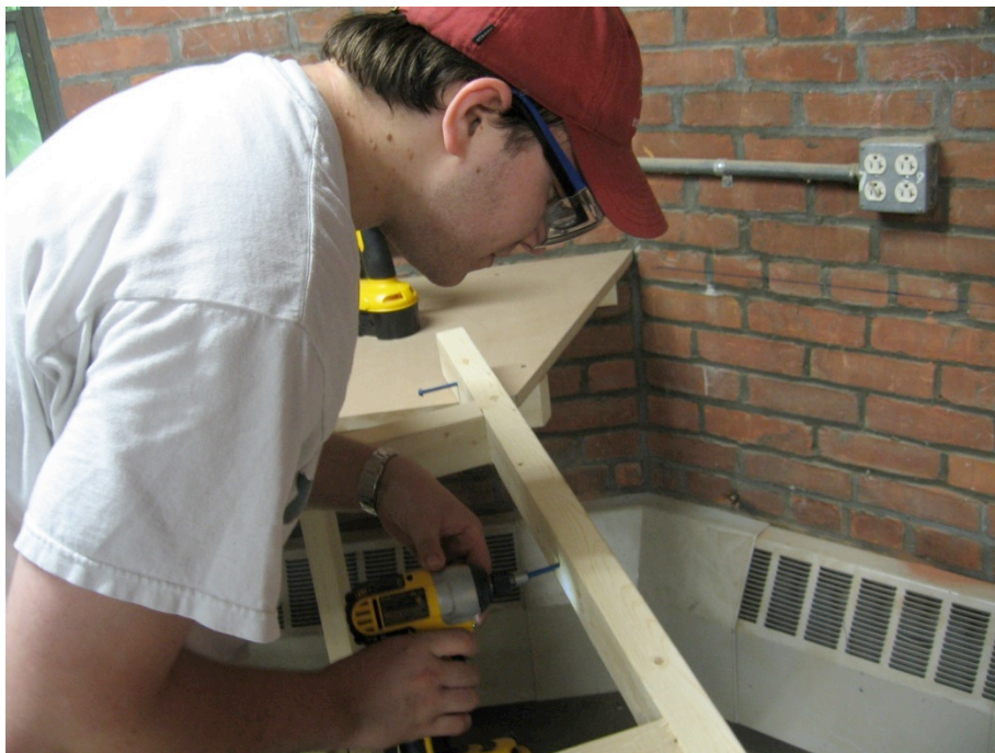
Paul assembles a frame using the new impact driver.
