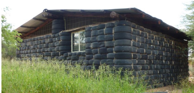
Figure 15. A Building Made from Tires at the HRDC
