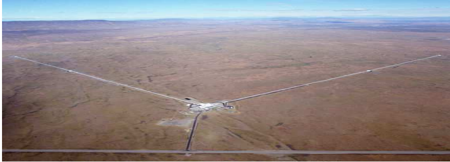
Figure 12: LIGO Hanford, Washington. Each tube is about 2km long.
