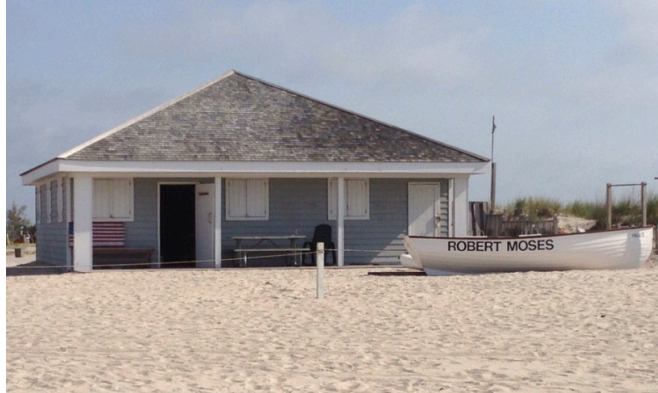
Figure 22 Field 3 Bathhouse, Robert Moses Park, Long Island, New York
