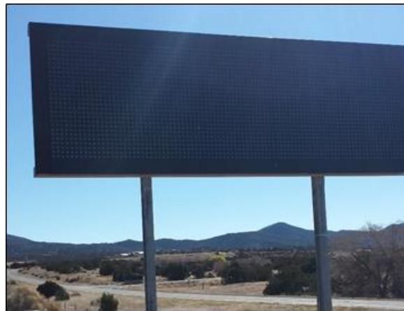
Figure 16. Roadside Dynamic Message Sign
