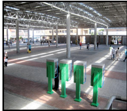
Figure 21: Covered Market Square (view from building B)
