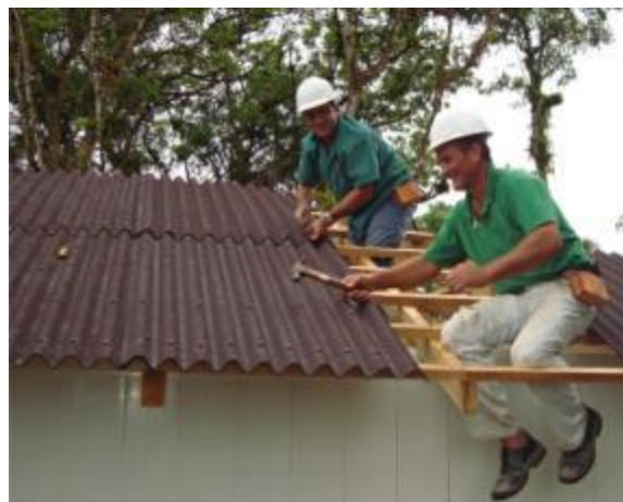
Figure 20: PVC Panel Roofing
