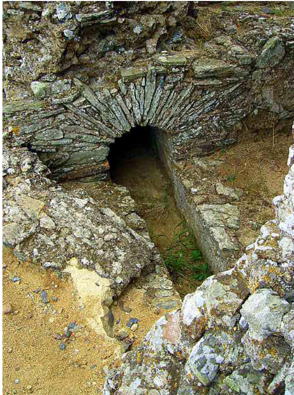
Figure 14: The Sboccho portion of a Fognatura system
