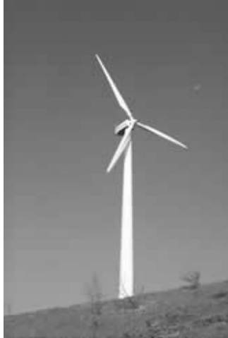
Figure 11: Horizontal Axis Turbine [13]
