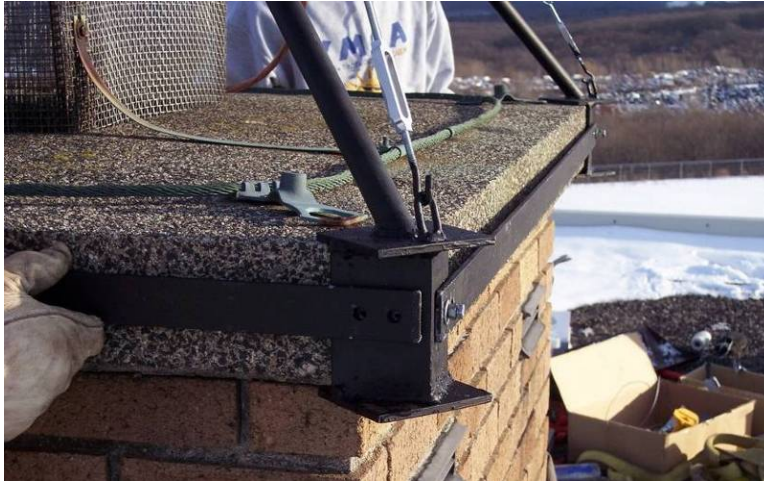
Figure 32: Corner Bracket and Braces Being Installed
