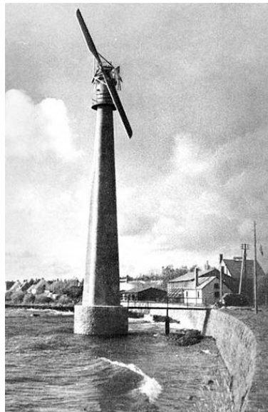
Figure 5: Smidth's Two Bladed DC Turbine [8]
