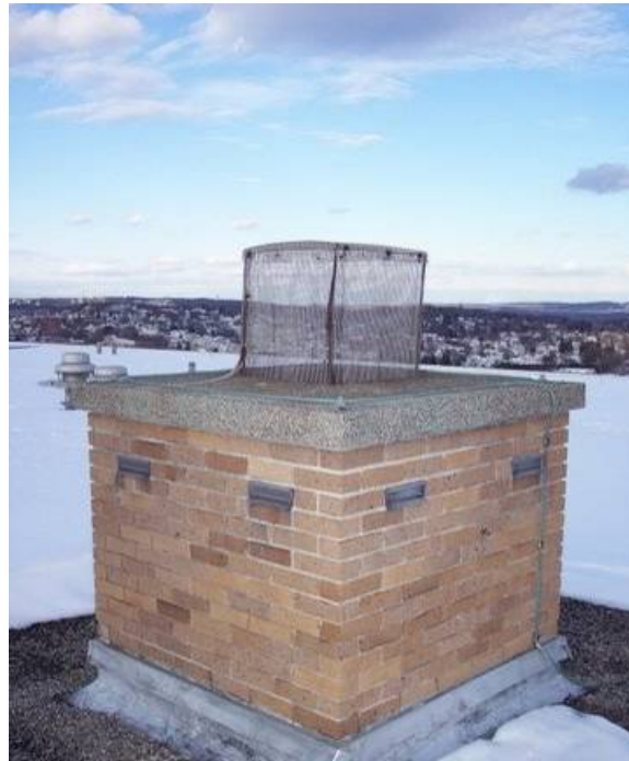
Figure 23: Existing concrete and brick chimney atop Holy Name (4' x 4' x 5')
