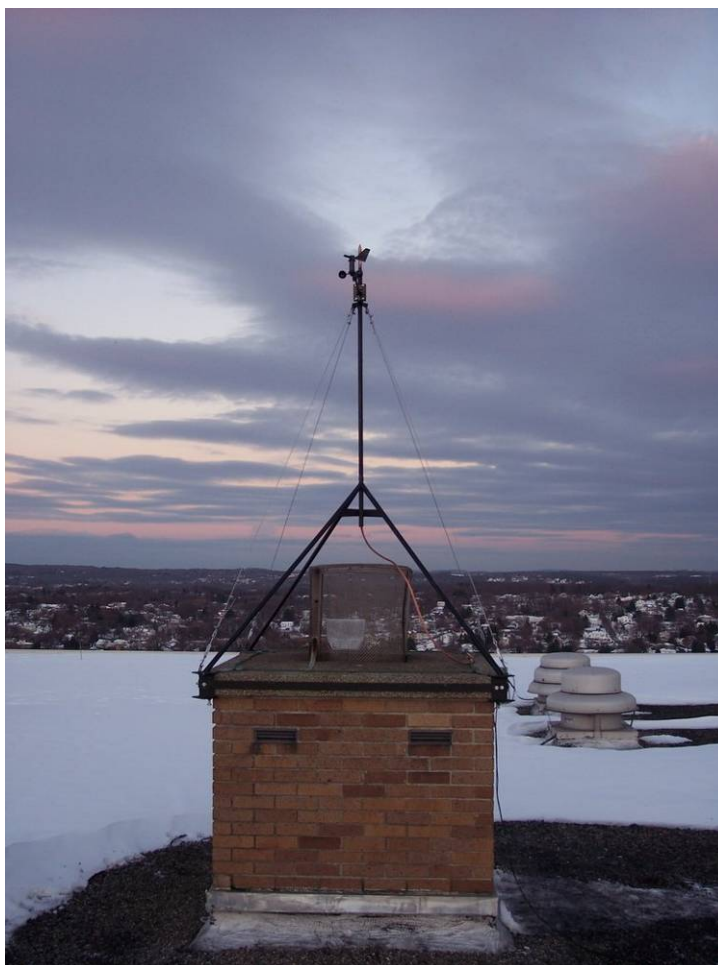
Figure 35: Tower Fully Installed
