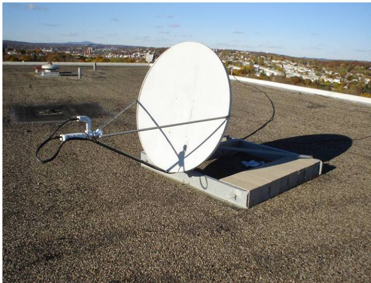
Figure 24: Satellite dish mounted on cinder block platform atop Holy Name
