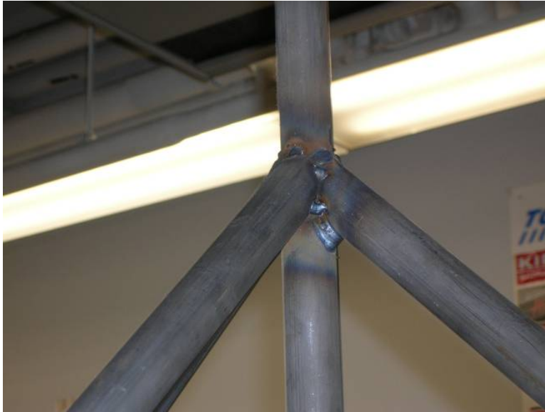
Figure 27: Close Up of Supporting Pole Connection
