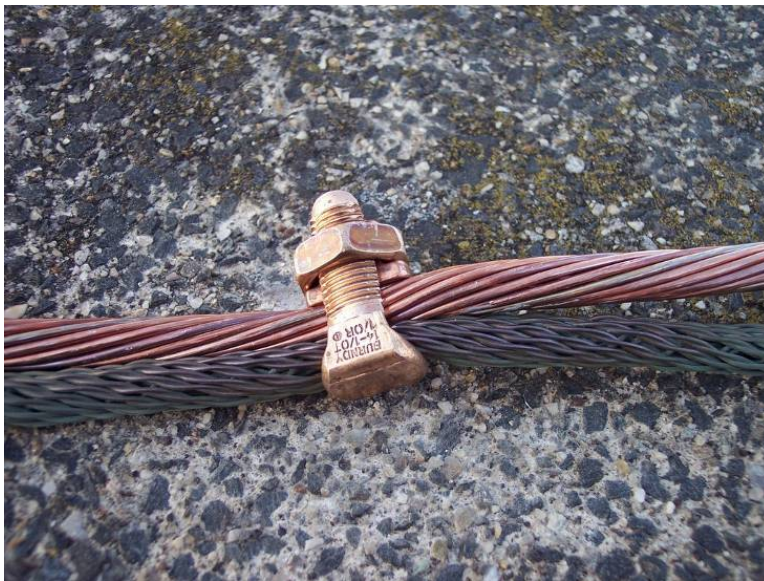
Figure 30: Lightning Protection Connection to Existing System
