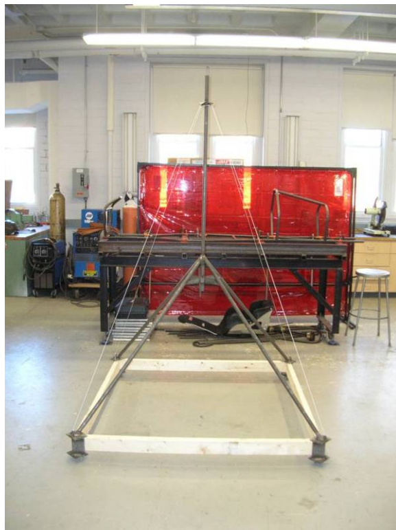
Figure 28: Tower Completed and Ready for Paint
