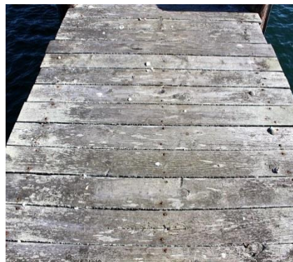
Figure 45: Rotting decking
