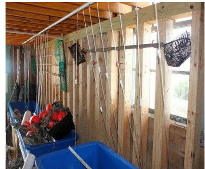
Figure 74: Rebuilt wall frame in Shellfish Lab
