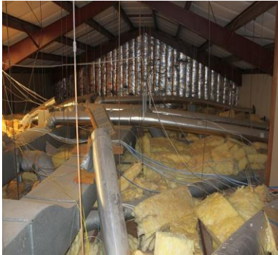
Figure 24: Messy attic at PLUS
