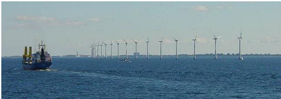
FIGURE 32: MIDDELGRUNDEN OFFSHORE WIND PARK (MIDDELGRUNDEN, DENMARK)
