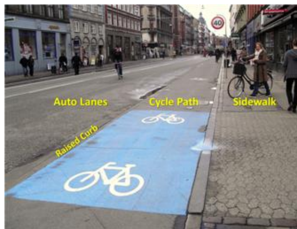
Cycle path separated from moving auto lanes by a raised curb, which may or may not be to the right of parked cars
