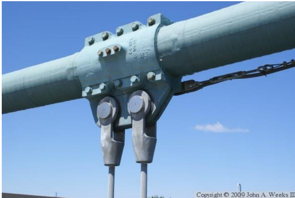
Figure 43: Example of Arch-Cable Connections
