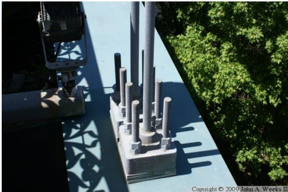
Figure 44: Example of Cable-Girder Connection
