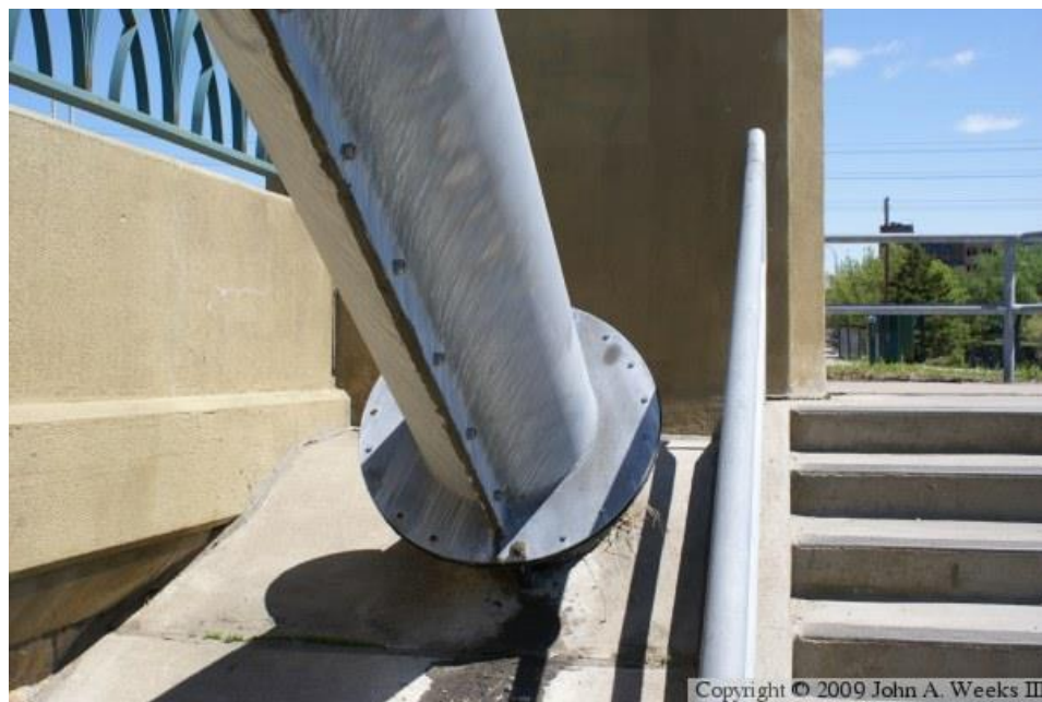
Figure 45: Example of Arch-Foundation Connection
