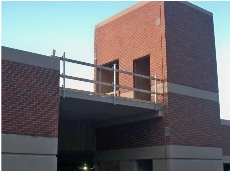
Figure 25: Here the bridge decking will meet the Parking Garage
