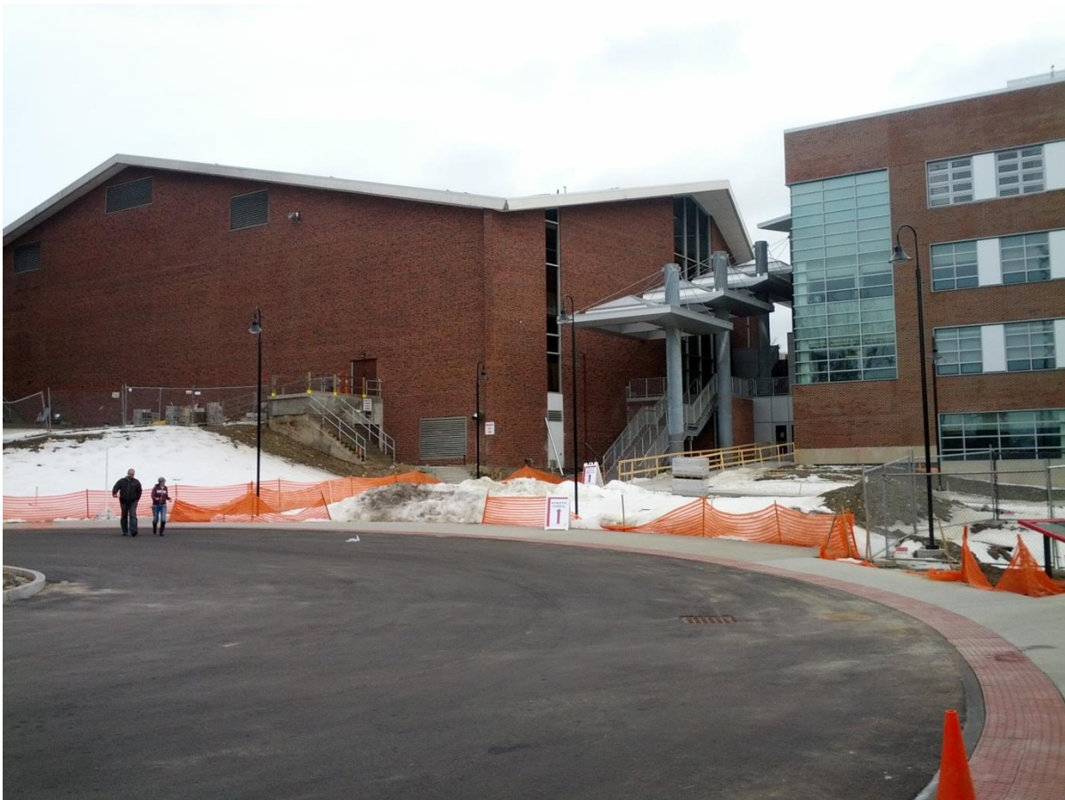
Figure 21: Looking Towards the Loading Dock
