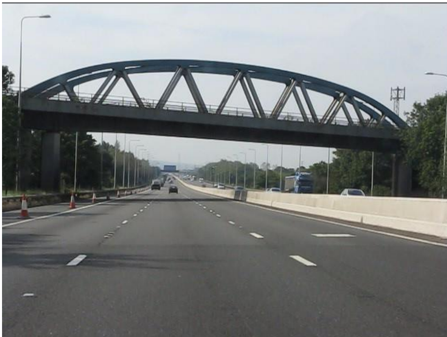
Figure 6: Hallen Bridge over the M5 Motorway in Great Britain
