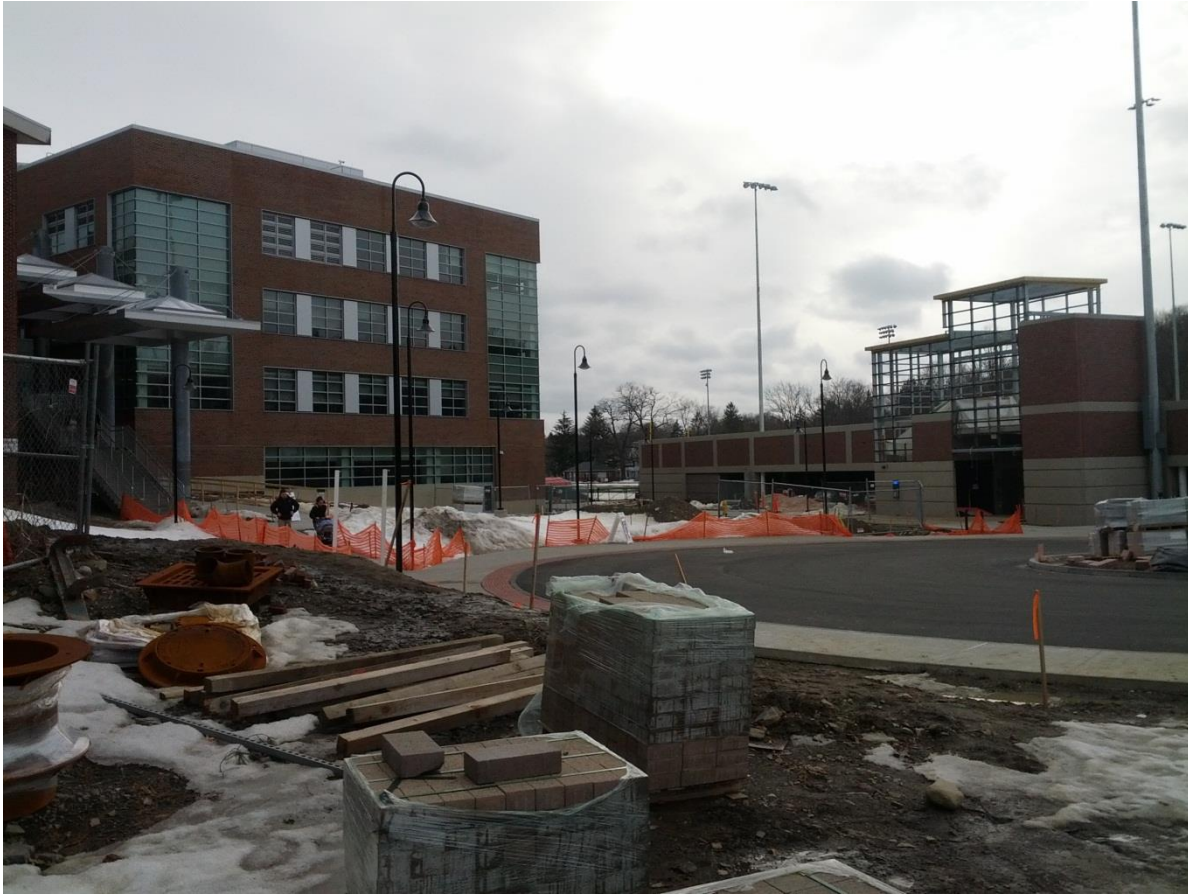
Figure 22: looking Towards the Parking Garage
