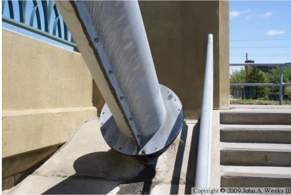
Figure 45: Example of Arch-Foundation Connection
