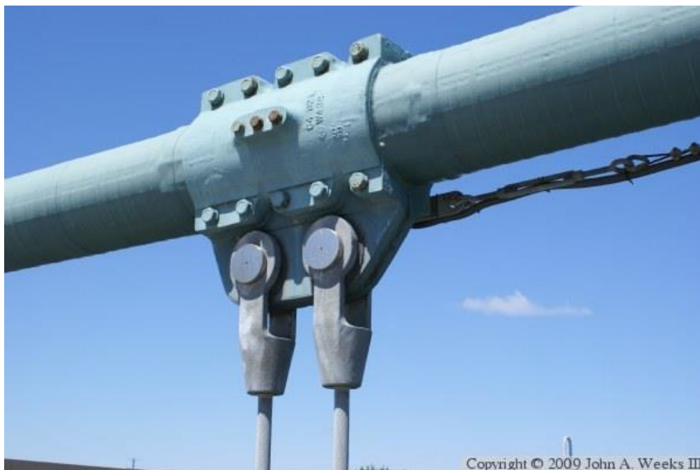
Figure 43: Example of Arch-Cable Connections
