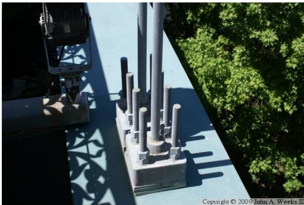
Figure 44: Example of Cable-Girder Connection
