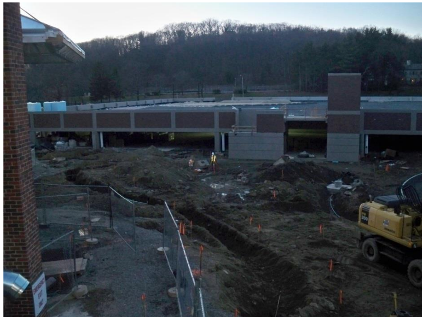
Figure 27 : View From Harrington, overlooking the construction Area, the Parking Garage is in the Distance
