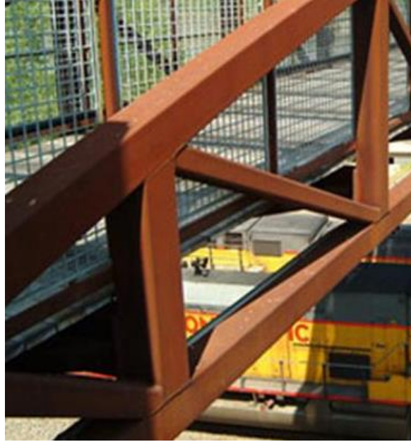
Figure 38: Typical Welded steel Connection
