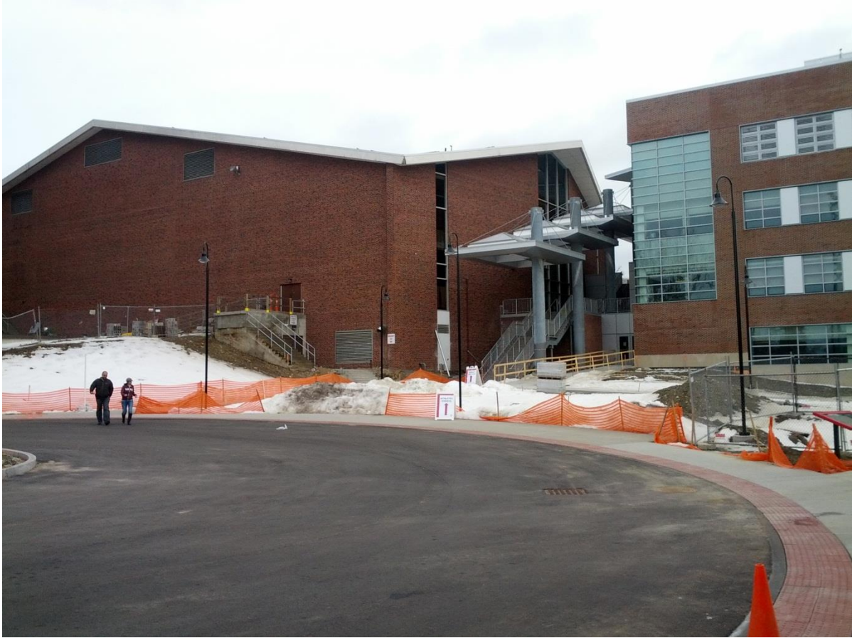
Figure 21: Looking Towards the Loading Dock
