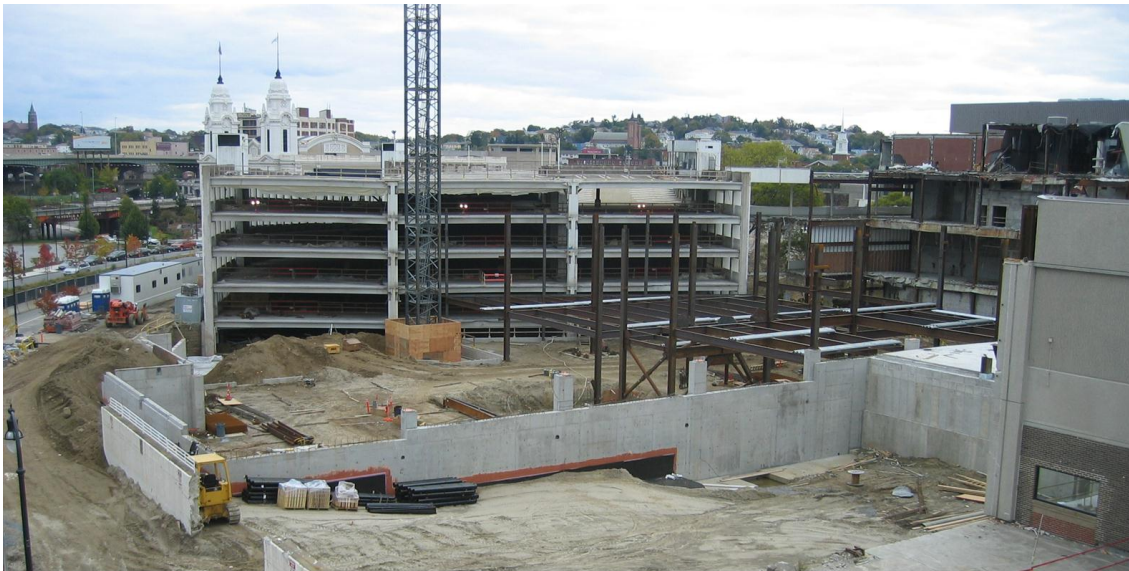
Figure 14 - Week 1 Progress Picture
