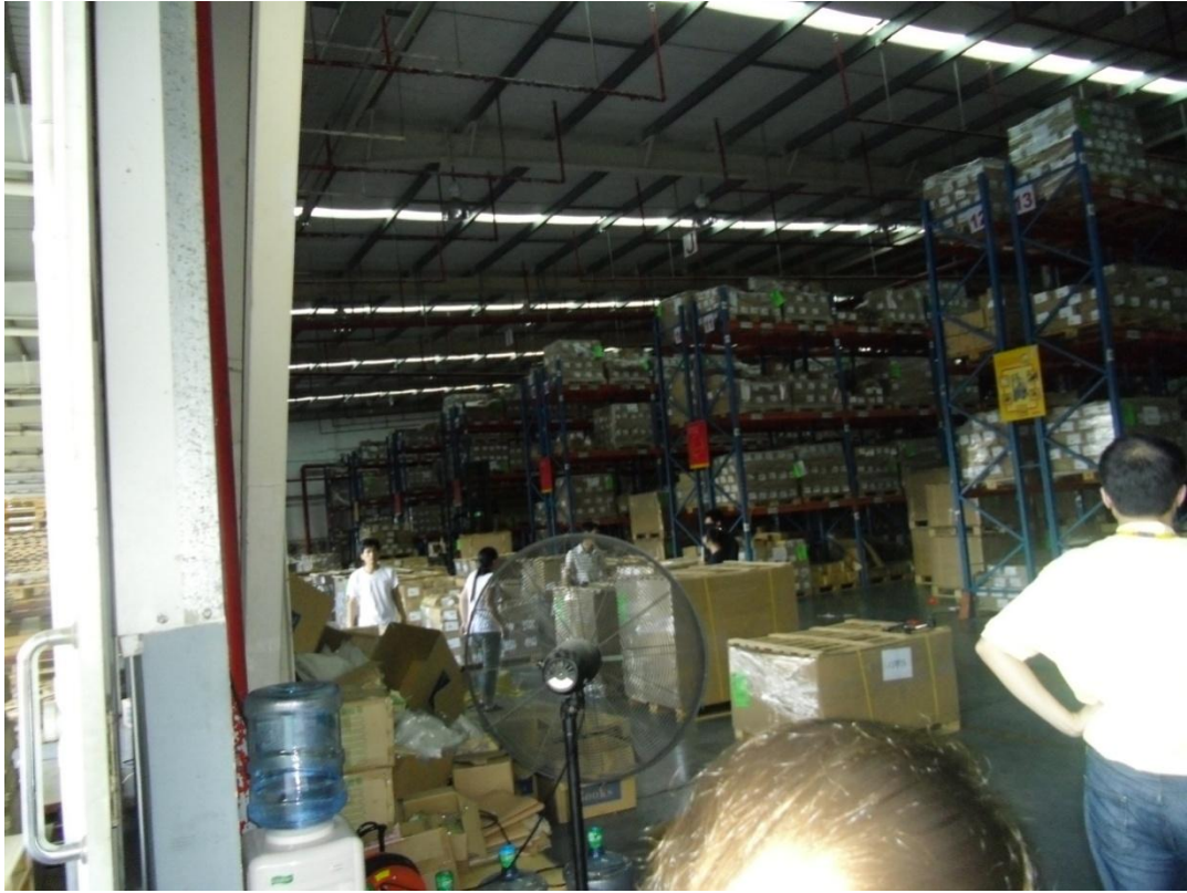
Figure 18: Example of Racking System 1
