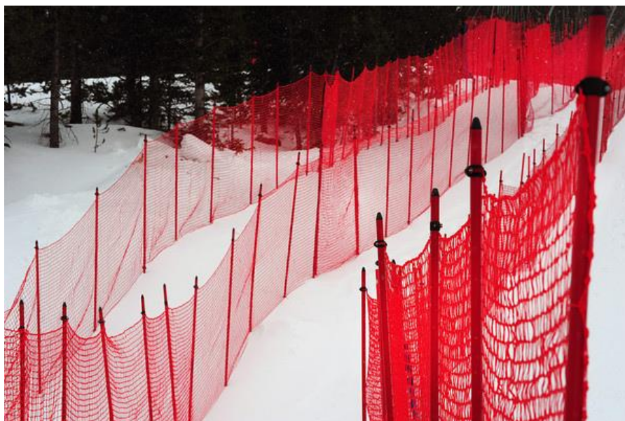
Figure 3: B-net deployed in three layers
