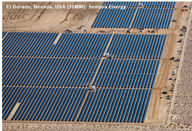
Figure 35 - 10 MW facility at El Dorado, Nevada. 151
