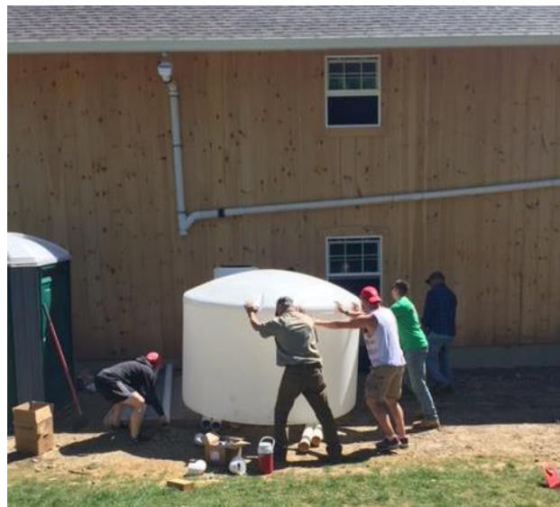
Figure 20: Construction Day 2: Moving Barrel into Place Image Source: Lisa Stoddard
