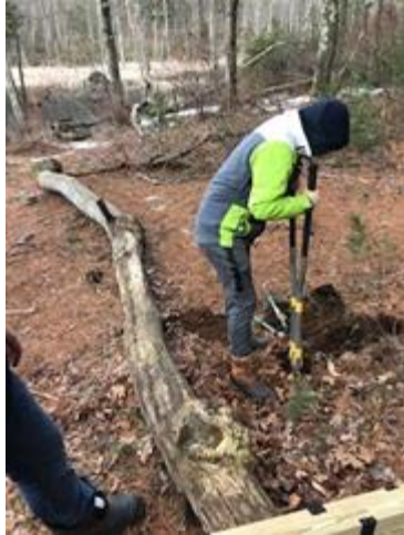
Figure 30. Digging of Post Holes
