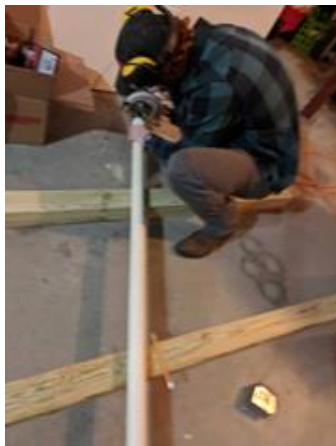
Figure 26. Cutting of PVC Pipes
