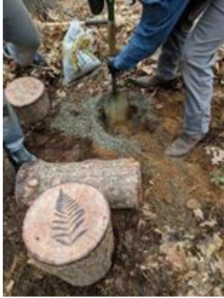
Figure 21. Holes for the logs
