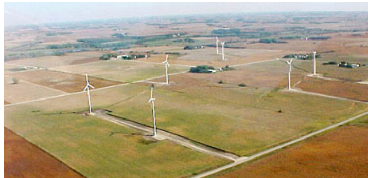
Figure 15: Top of Iowa Wind Farm
