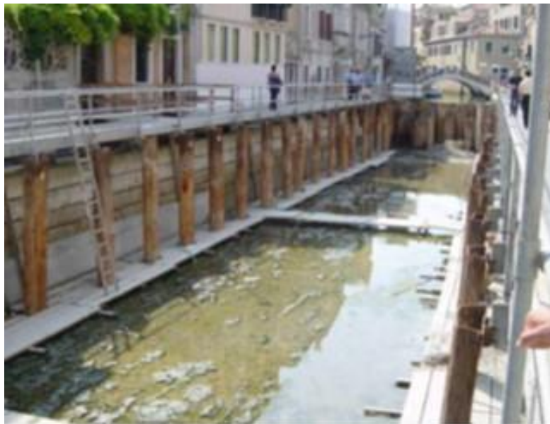
Figure 52: A canal wall undergoing repairs.
