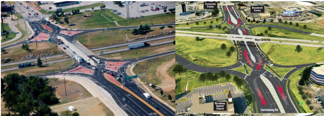
Source: 13 (MnDOT Construction Project: Diverging Diamond Interchange)
