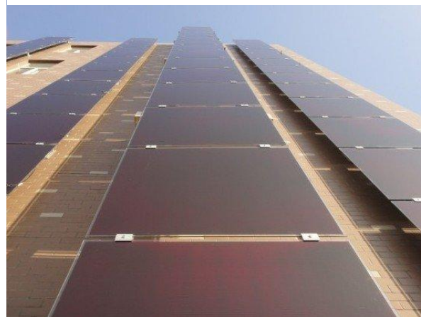
Source: 4 (Building Integrated Photovoltaics)
