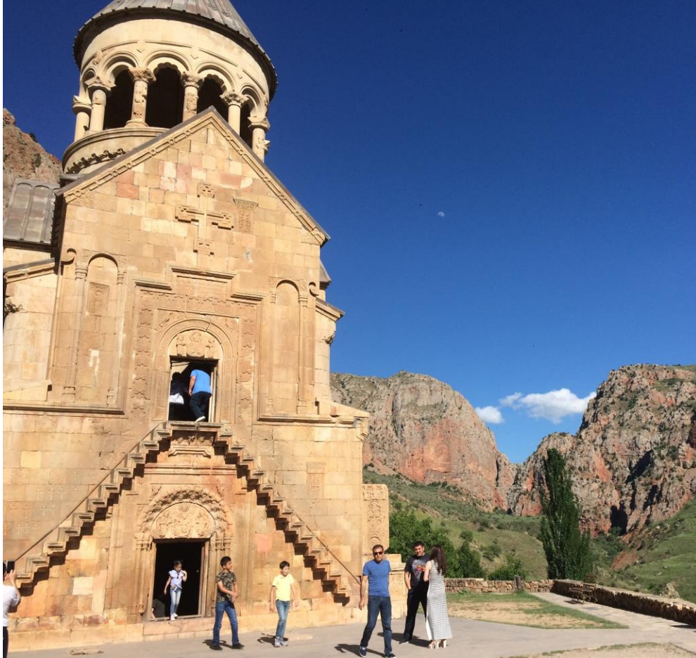
Figure 6: Entrance to the second floor of the Noravank Monastery
