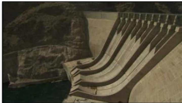
Figure 87: Karakaya Spillway, Turkey (Karakaya Dam, 2015)
