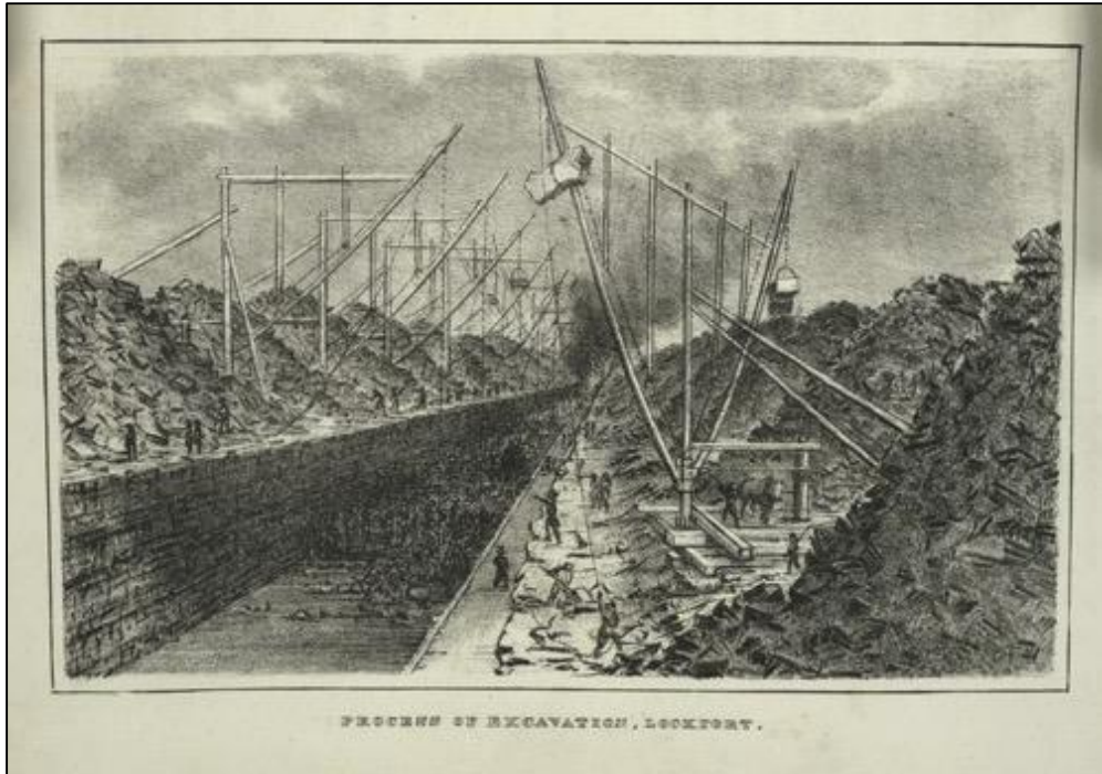
Figure 1: Makeshift pulleys and early machinery involved in 1800s canal building (Root, 2015)
