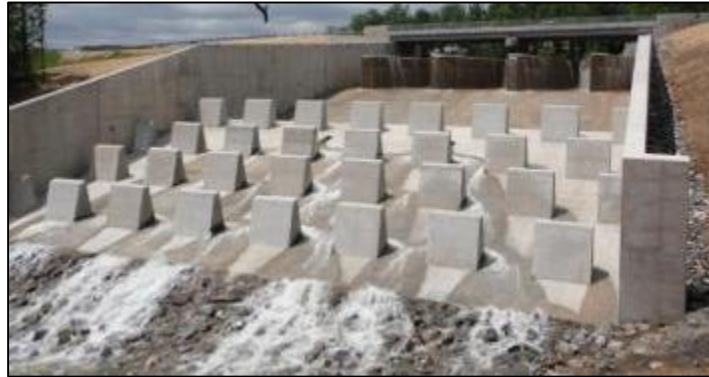
Figure 68: Open chute spillway with large baffle blocks (C. William Hetzer, Inc., 2012)
