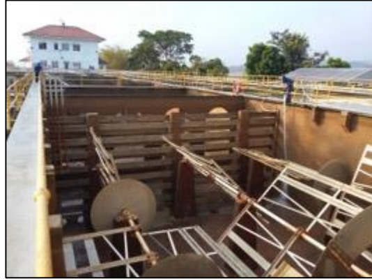
Figure 46: Flocculation Propellers
