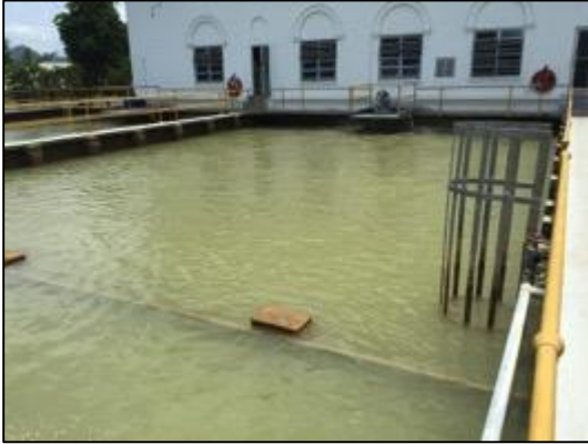
Figure 45: Flocculation Basin
