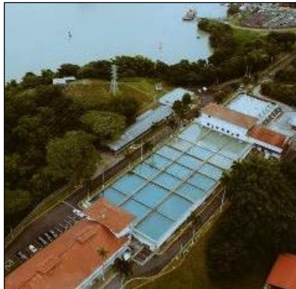
Figure 37: Miraflores Water Treatment Plant (Canal de Panamá, 2015)
