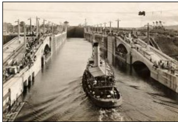
Figure 34: Gatún Tugboat making the first pass through the Gatun Locks (Smith, 2014)
