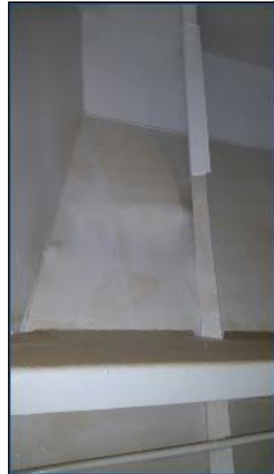
Figure 62: R-GUÍA tank inspection 7-7
