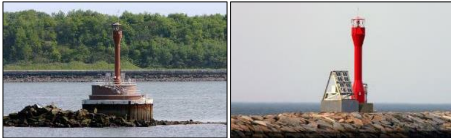
Figure 30: Deer Island Light and Cape Cod Canal Breakwater Light (Rowlett, 2015d)
