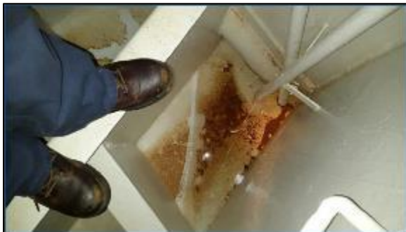
Figure 58: R-GUÍA tank inspection 3-7
