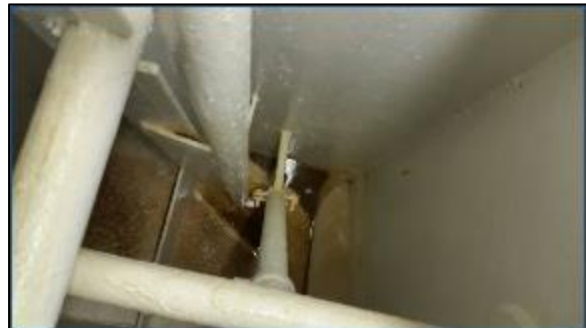
Figure 57: R-GUÍA tank inspection 2-7
