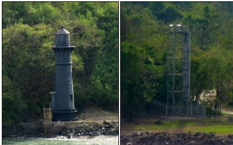
Figure 26: Balboa Southbound Rear Range Tower (Rowlett, 2014b)
