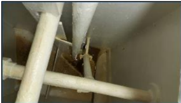
Figure 56: R-GUÍA tank inspection 1-7
