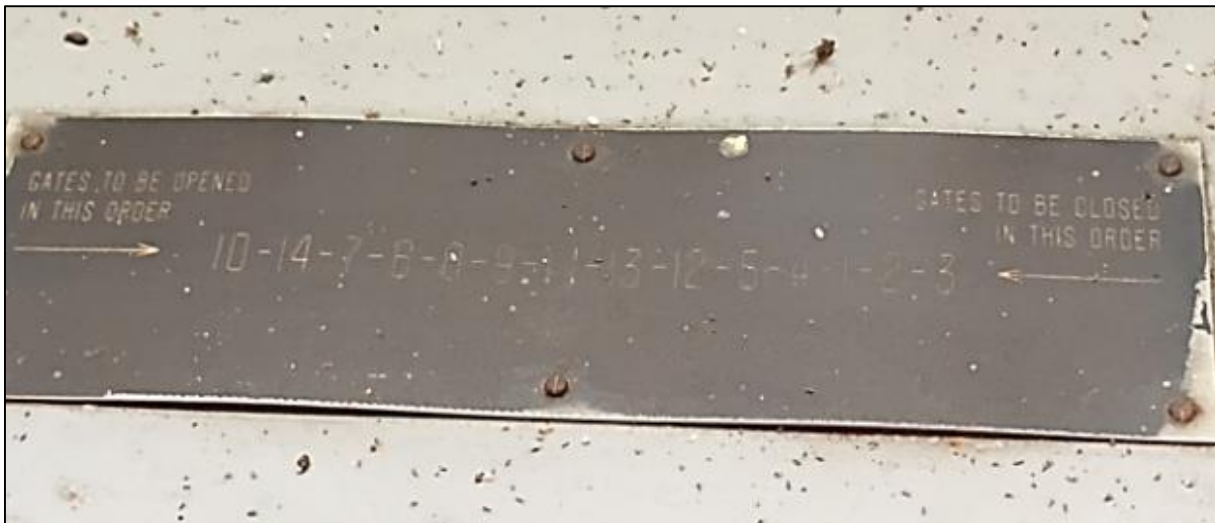
Figure 77: Order of opening Gatun Spillway gates: 10-14-7-6-8-9-11-13-12-5-4-1-2-3. The order is reversed for closing the gates.
