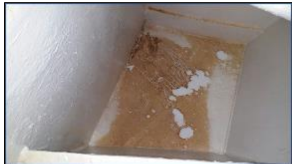
Figure 59: R-GUÍA tank inspection 4-7
