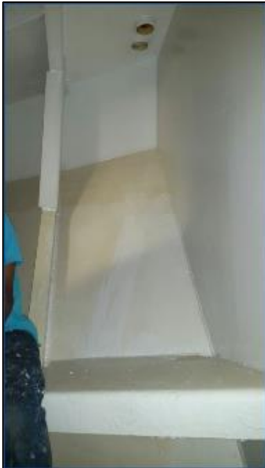
Figure 60: R-GUÍA tank inspection 5-7
