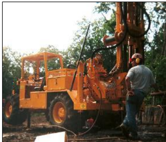
Figure 80: Machinery used for borehole drilling (Raimonde Drilling Corporation, 2015)
