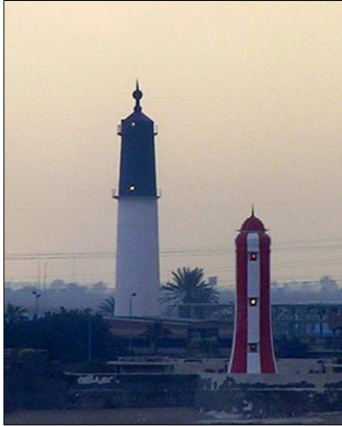
Figure 22: Great Pass Range Lighthouses in Alexandria, Egypt (Rowlett, 2015a)
