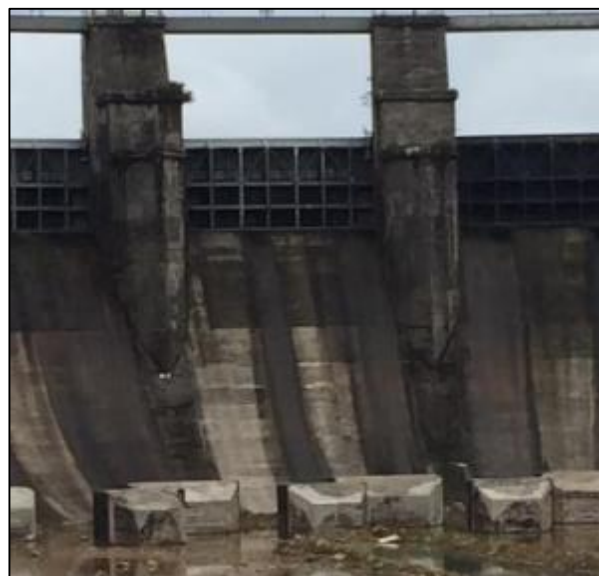
Figure 74: Baffle blocks of the Gatun Spillway and basin
