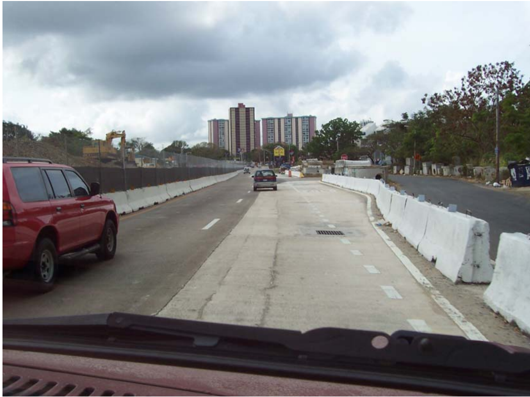
Figure 70: 181 South Heading to Park Gardens Intersection
