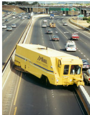
Figure 60: Zipper Machine moving two lanes
