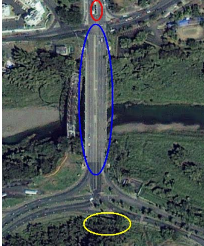
Figure 36: Via Encantada Intersection
