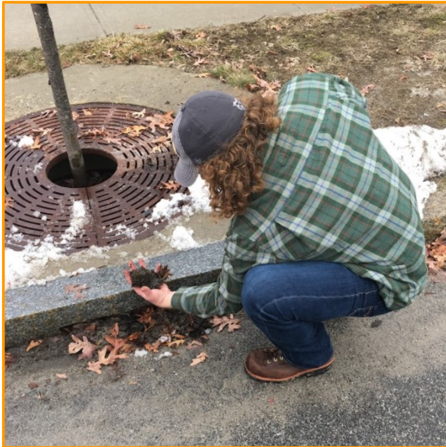
Blayne Merchant investigating a clogged tree box filter in Worcester.
