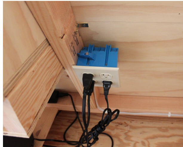
Figure 24 – Dual-Receptacle Box
