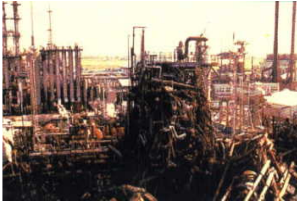
Figure 2-1: Devastation in Seveso
