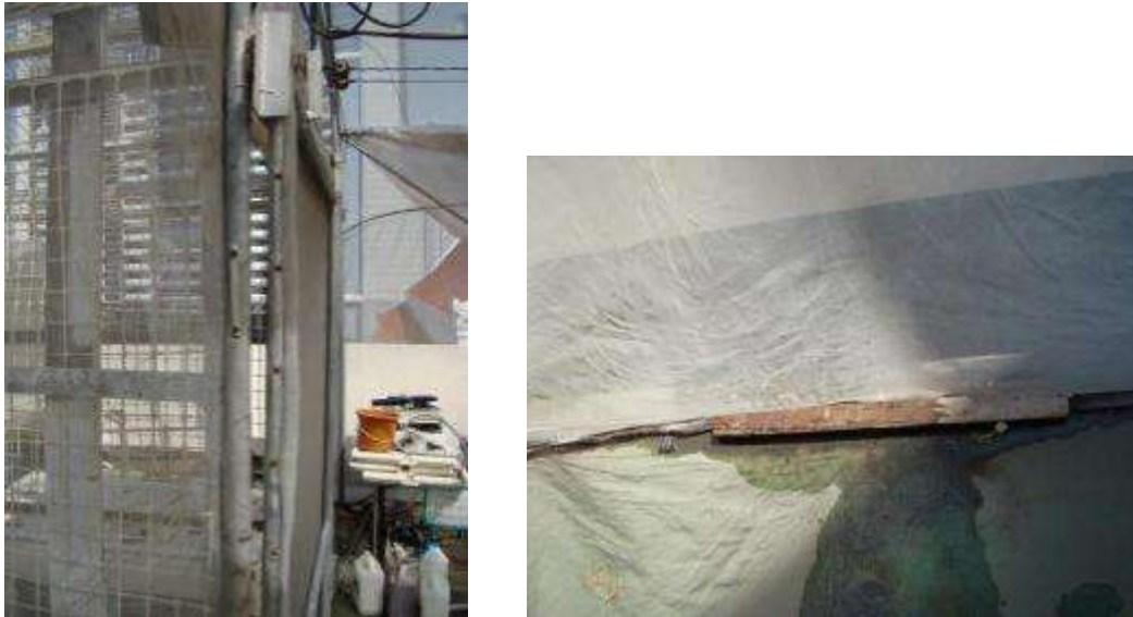
FIGURE 14: ACCESS POINTS IN THE DOOR (LEFT) AND NETTING (RIGHT)
