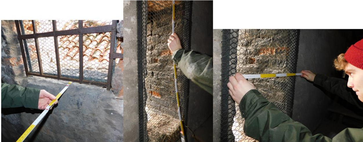
Figure 20 - Measuring interior window dimension, from left to right: depth, height, and width
