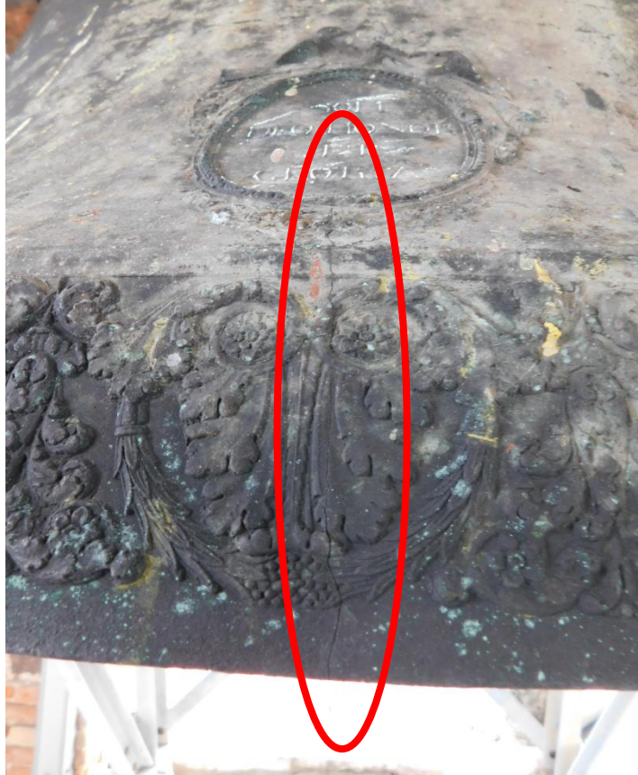
Figure 71 - Crack in Bell 3 of Frari
