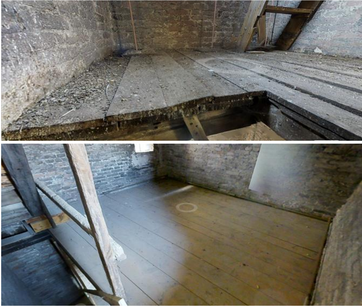
Figure 19 - Top: 1 Ranking (worst possible) for Landing Cleanliness, Bottom: 4 Ranking (generally clean) for Landing Cleanliness
