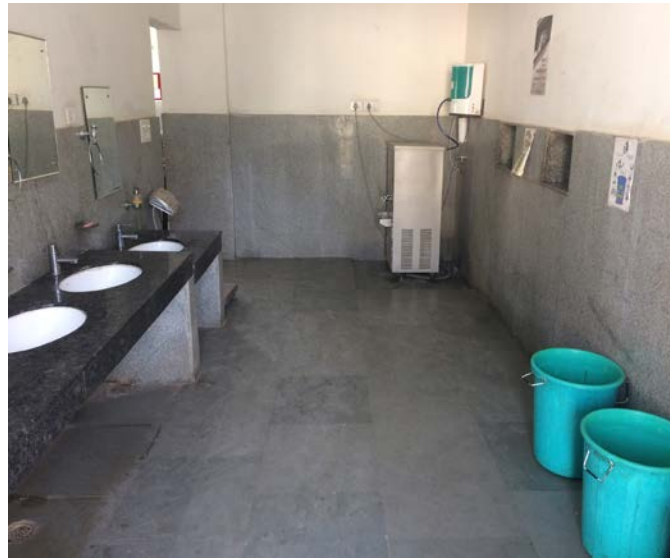
Figure 3: The waste disposal area at D2 mess
