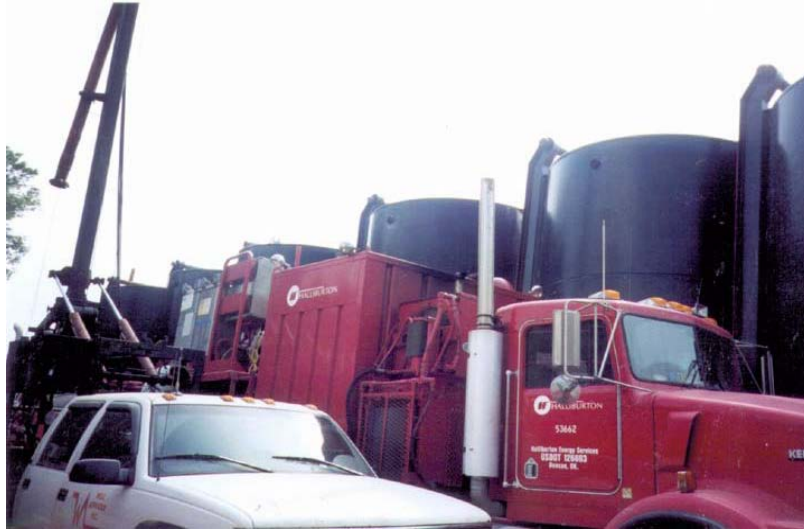
Figure 3.1: The fracturing fluid (water and chemical additives) is stored commonly on site in large, upright storage tanks. These tanks can contain anything from water, wastewater, or chemical additives. xxxix
