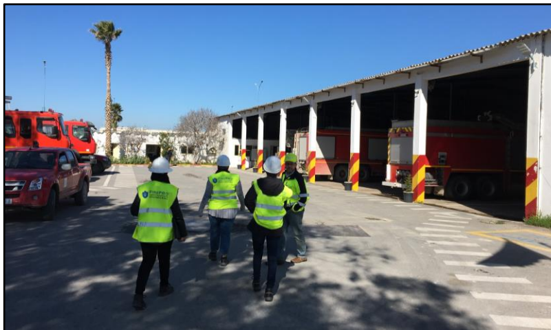
Figure 43: Entrance to the fire department at OCP, four fire trucks are on site
