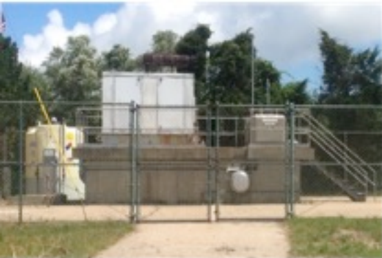
Elevate Utilities and Generator
