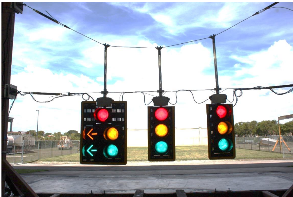
Figure 2-13 – Modified traffic light assembly (5% sag, 7 feet distance between catenary and messenger load cell, 125% of standard messenger wire pre-tension)
