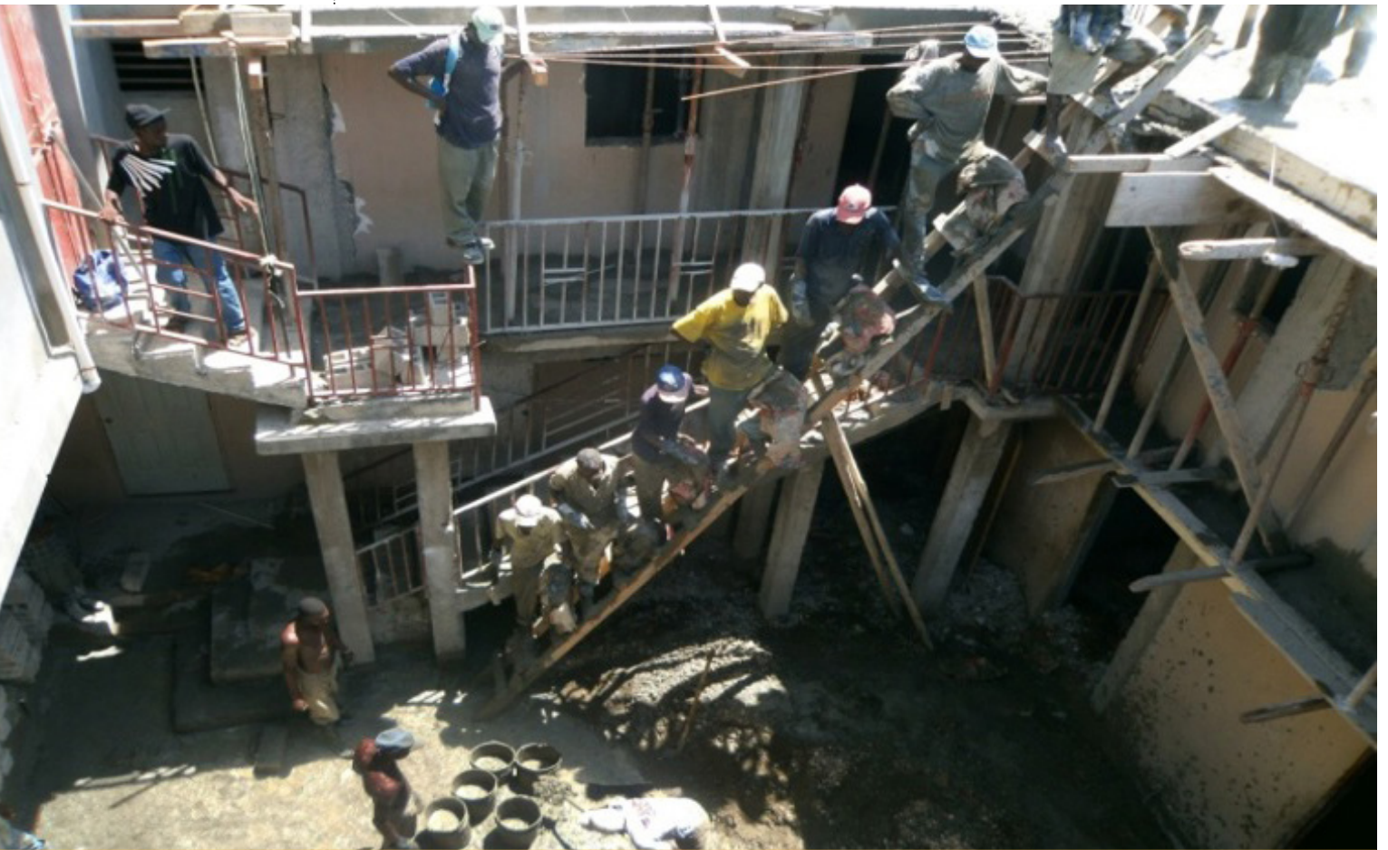
World Concern-Haiti School-shelter retrofiting Photo: WCDO
