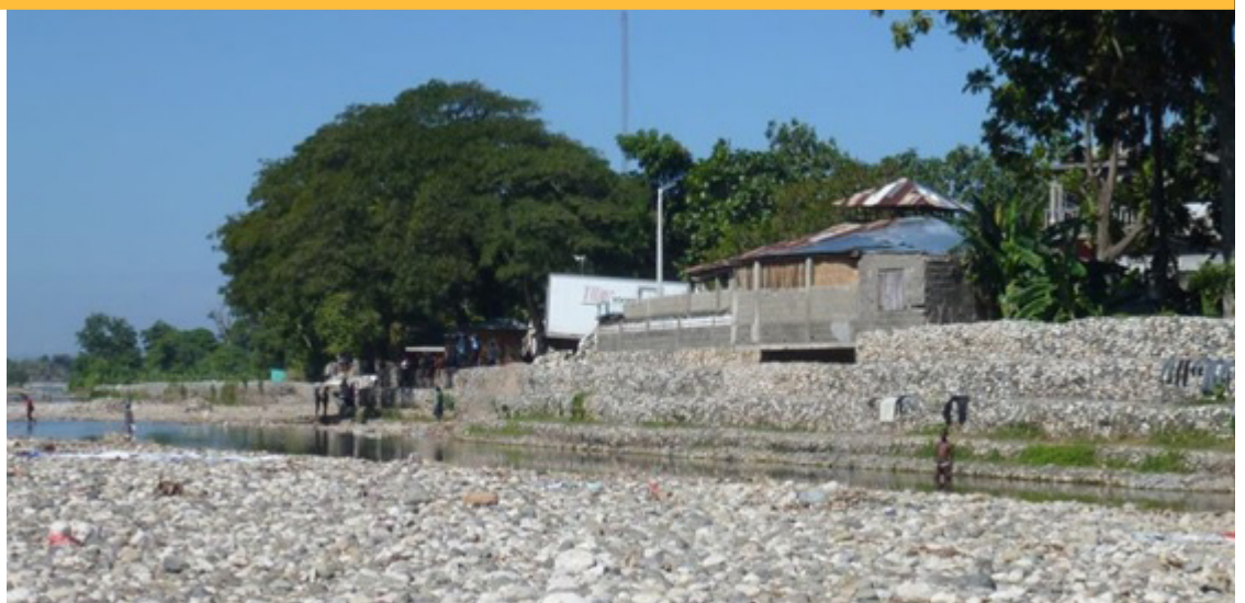
World Concern Haiti Gabions completed Photo: WCDO
