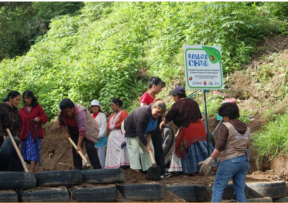
CRS Quetzaltenango- Guatemala-Women building public infrastructure Photo: CRS
