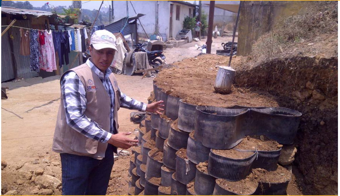
PCI Mixco-Guatemala- Retaining wall using tires Photo: PCI
