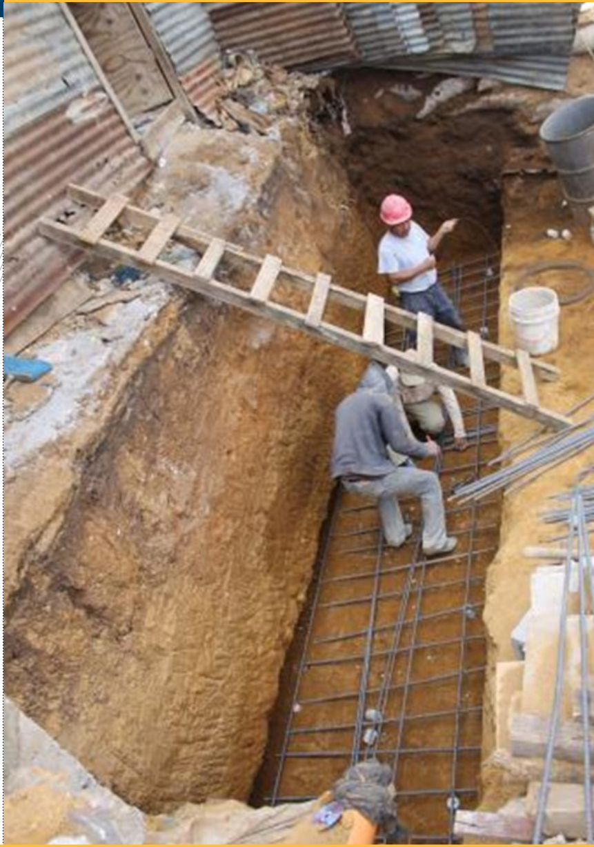
PCI Mixco-Guatemala- Building retaining walls Photo: PCI
