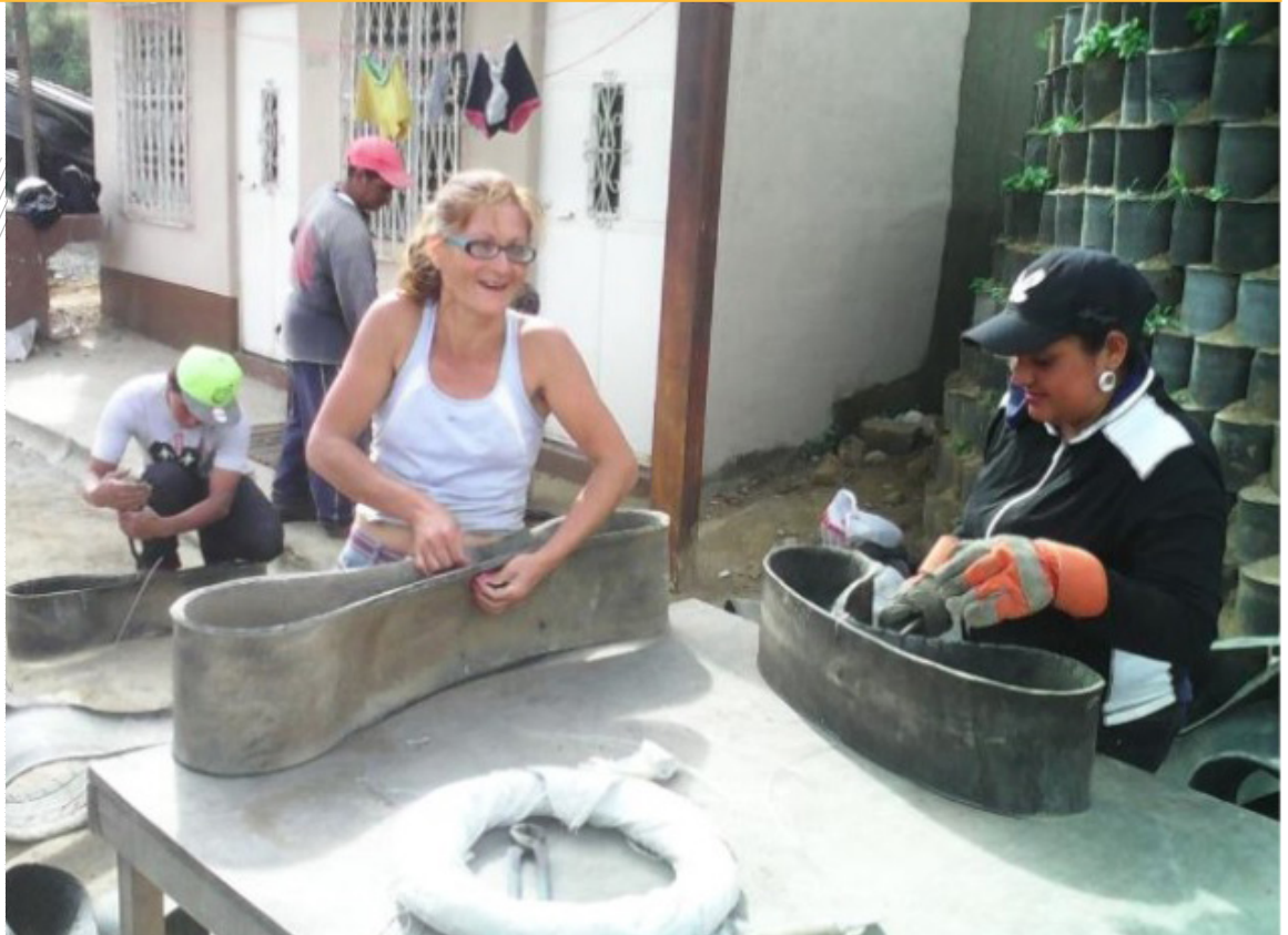
PCI Mixco-Guatemala- Empowered women retaining walls Photo: PCI
