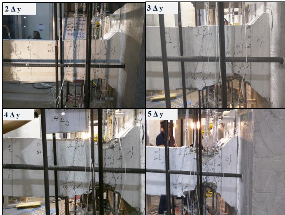
Figure 4-7 Plastic hinge damage at different displacement levels.
