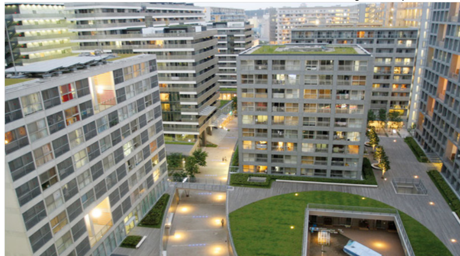
Shinonome Canal Court Tokyo, Japan
