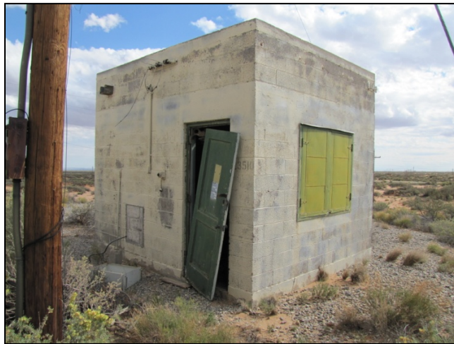
Figure 36. Camera Building, Tare Site, 2016
