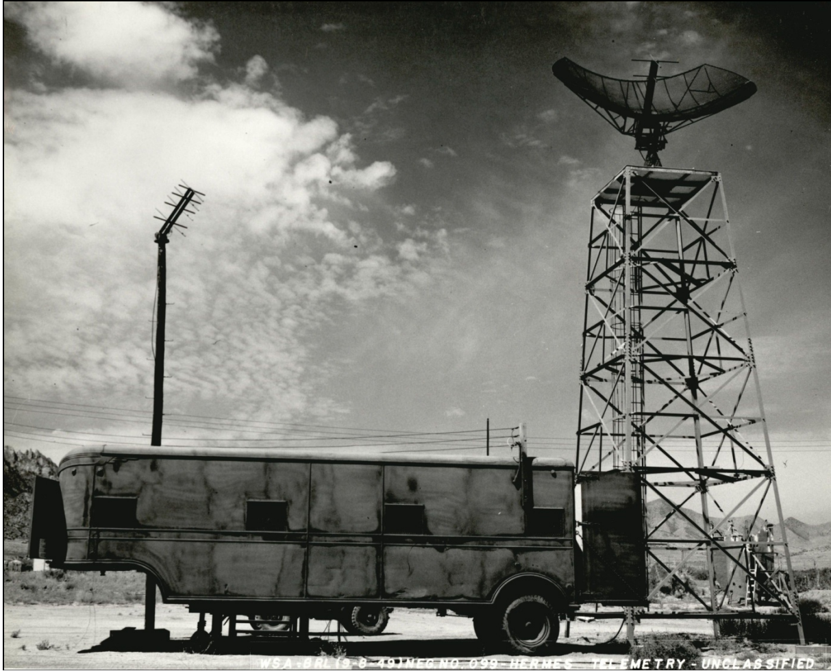
Figure 5. Telemetry Station at WSPG, 1949 (White Sands Museum Archives 06.003.028)
