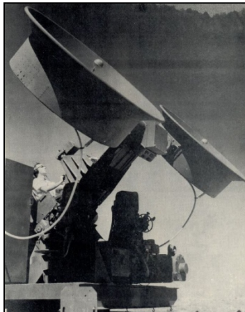
Figure 71. Velocimeter at WSPG (WSMR Picture Brochure, 1956)
