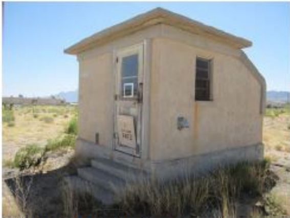
¾ view of the exterior, view southwest
