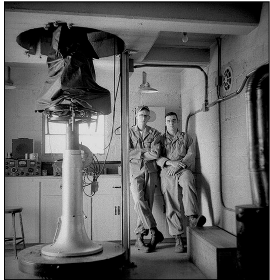
Figure 16. Cinetheodolite on hydraulic lift, 1955 (WSMR Museum Archives)
