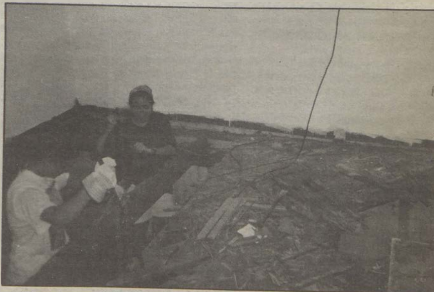
Members of Habitat for Humanity rebuild a termite-eaten floor.
