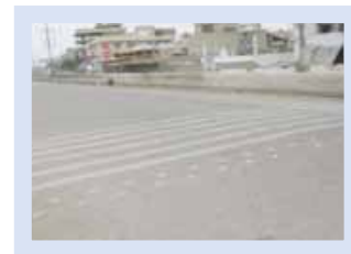
Fig. 3. Jinnah Bridge at Karachi Port was one of the first flyovers in the city and the high density of traffic injuries particularly of motorcyclists drew our attention to its inherent design flaws. In 2007, the surface treatment to enhance friction was done along with installation of speed reduction road furniture, with gratifying reductions of crashes reported over the next two years of observations.
