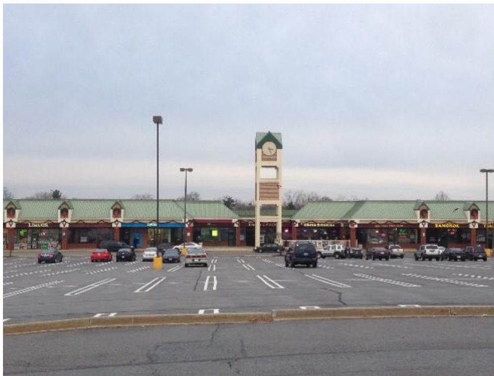
FIGURE 2 - WESTRIDGE SHOPPING CENTER, ROUTE 40
