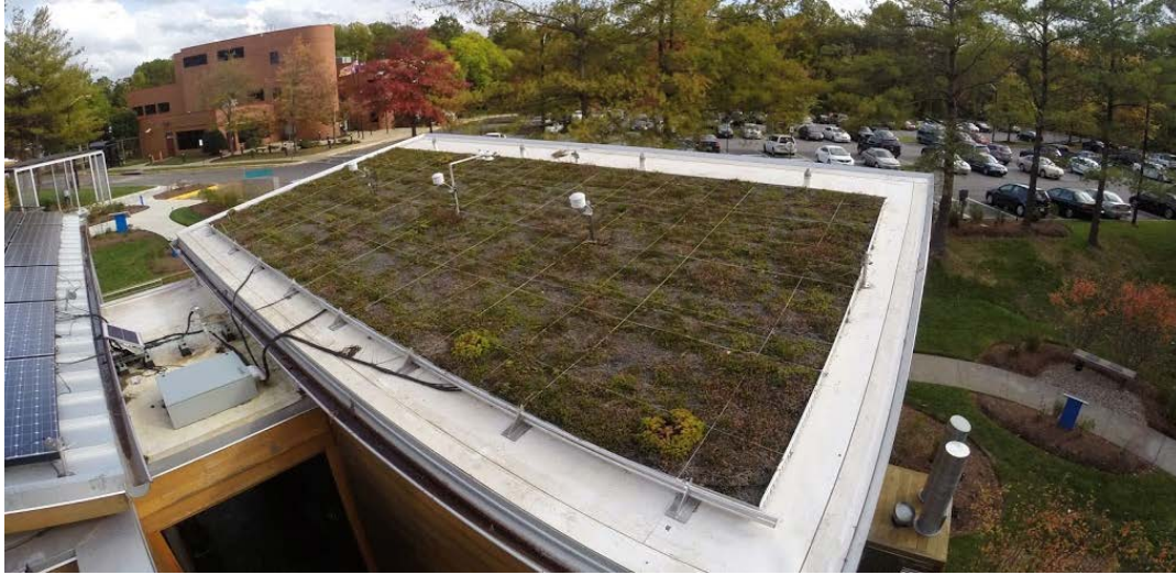
Figure 4-3 WaterShed's extensive green roof sits upon a cool roof (TPO membrane).
