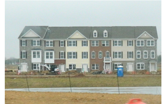
Site Visit Photos
