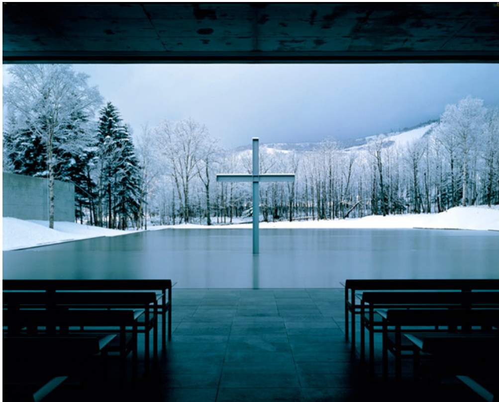
Figure 50: Church of Water- View Looking Out- Winter (Source: the-talks.com)
