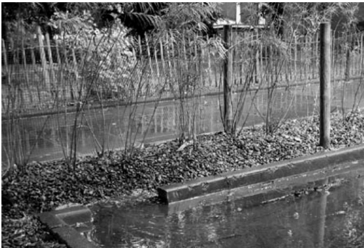
Figure 12: The combined stormwater detention BMP during a heavy storm. This image shows the inflow to the infiltration cell, with the detention cell below it (Debusk 2011)
