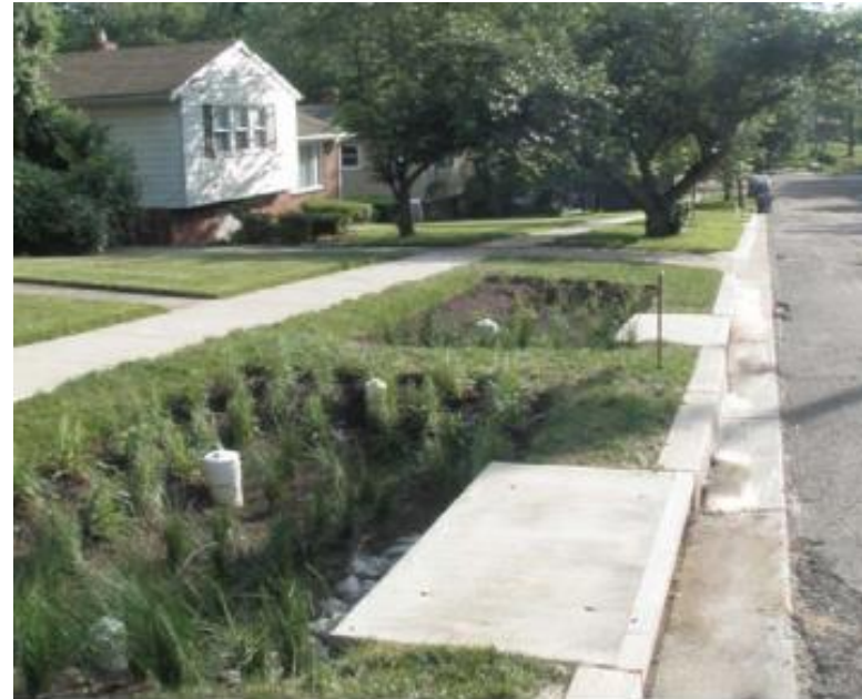
Figure 6.17. Bioretention Garden in Forest Estates (Montgomery County, MD 2012)
