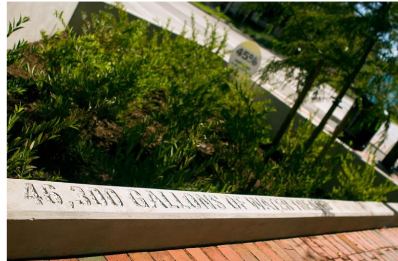
Figure 6.15. Bioretention Area with facts about stormwater along Bagby Street (Design Workshop 2014)
