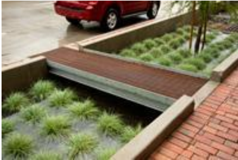
Figure 6.14. Bioretention Area along Bagby Street (Design Workshop 2014 )
