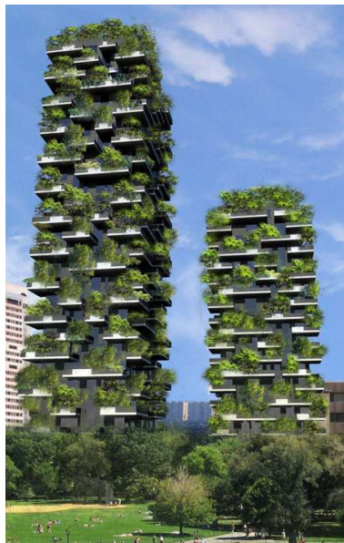
Figure 2 The Bosco Verticale project in Milan brings a vertical forest into two residential towers in the middle of the city (source: Nguyen Tan Tin, www.flickr.com )
