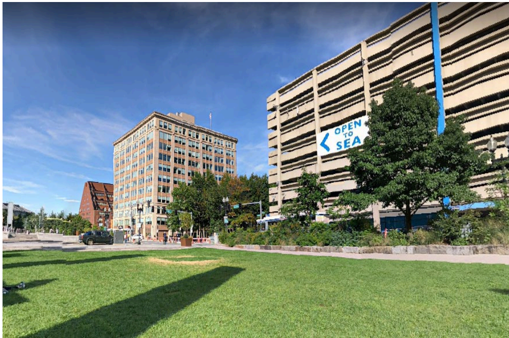
Figure 14: View of the Harbor Garage from the Greenway (source: Google Earth, edited by author)
