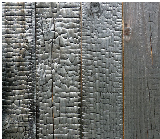
Figure 4 Shou sugi ban or charred wood facade (source: Wikimedia Commons)
