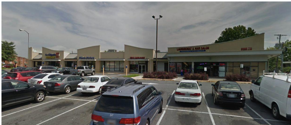
Figure 7: Street view of the the Site 3 shopping center
