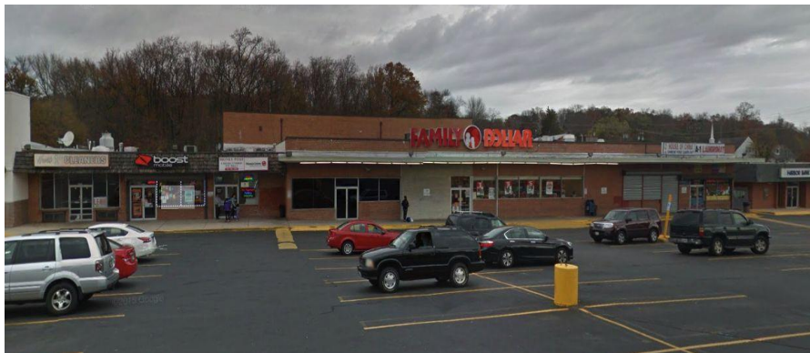
Figure 13: Street view of the Site 5 shopping center
