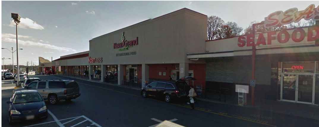
Figure 10: Street view of Site 4 shopping center
